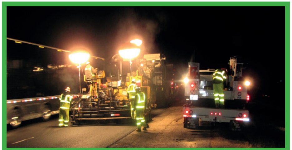
Road-surfacing at night close to live traffic.
