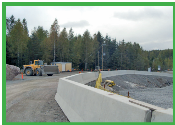
Edge Protection using precast structures.
