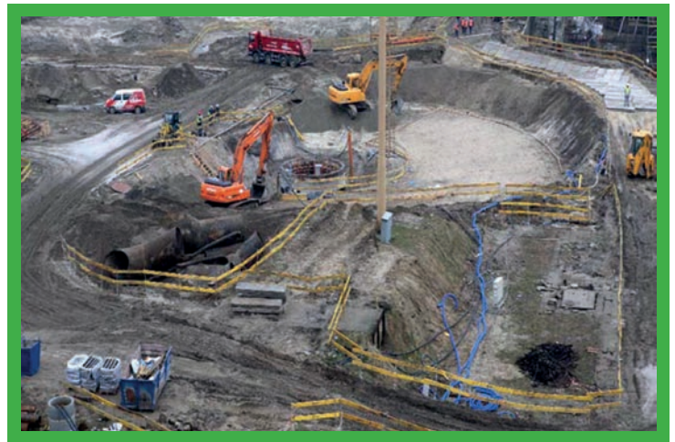
Transport systems at a construction site.
