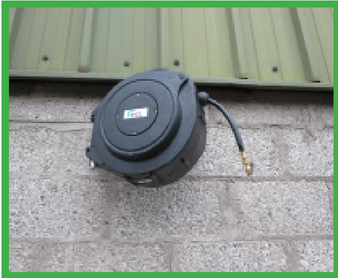
Best Practice example: To eliminate the risk of over inflation of tyres, tyre pressure is inputted remotely into a control unit. The 15 metre airline is then fitted to the vehicle (away from the control unit ) and a preset air pressure is used to inflate the tyre. Access to the control is restricted as users require access codes.
