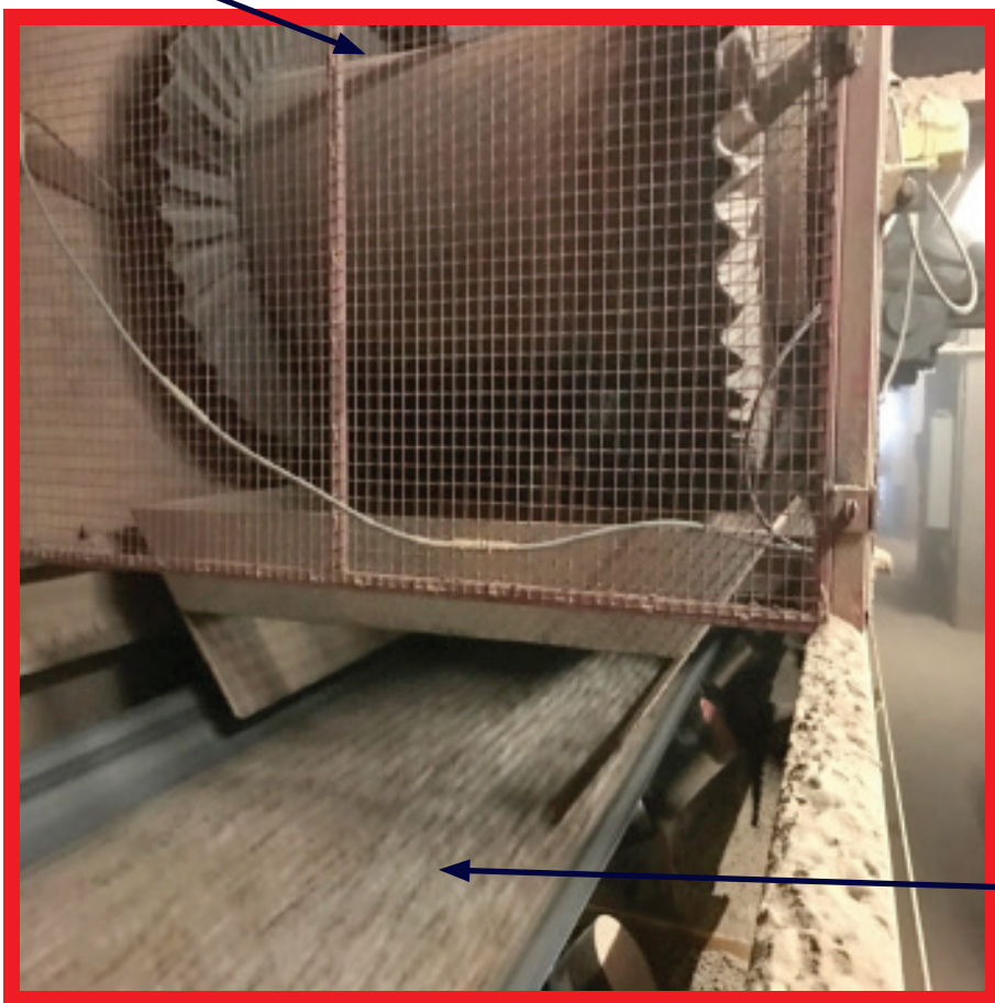
Contractors working on Feeder (which was off, but not isolated).
