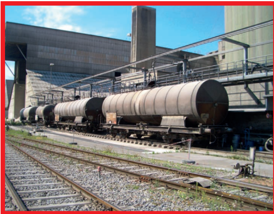
Incident 2011: A specialist contractor was engaged to carry out a general inspection of a rail wagon used for storing waste solvent. During this process the worker showed signs of being overcome by fumes - the person observing the work from outside entered the tank to assist and also experienced difficulties - a second observer activated the rescue plan and both men were safely removed and treated.
