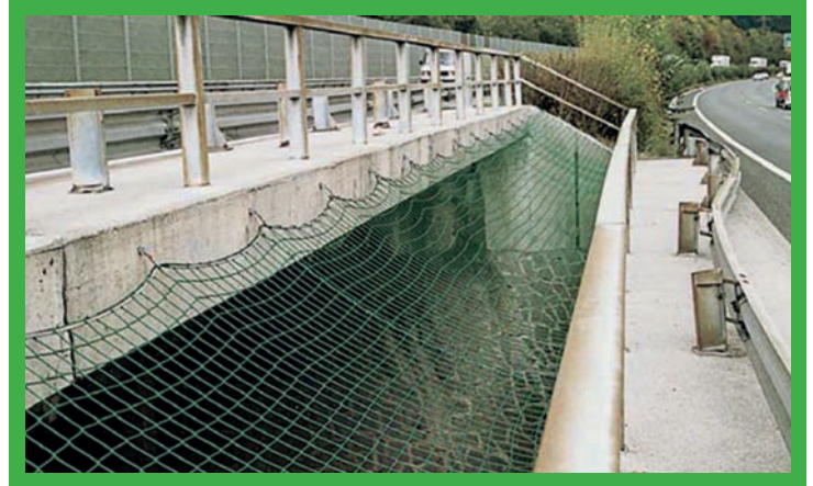
Safety Netting in place.
