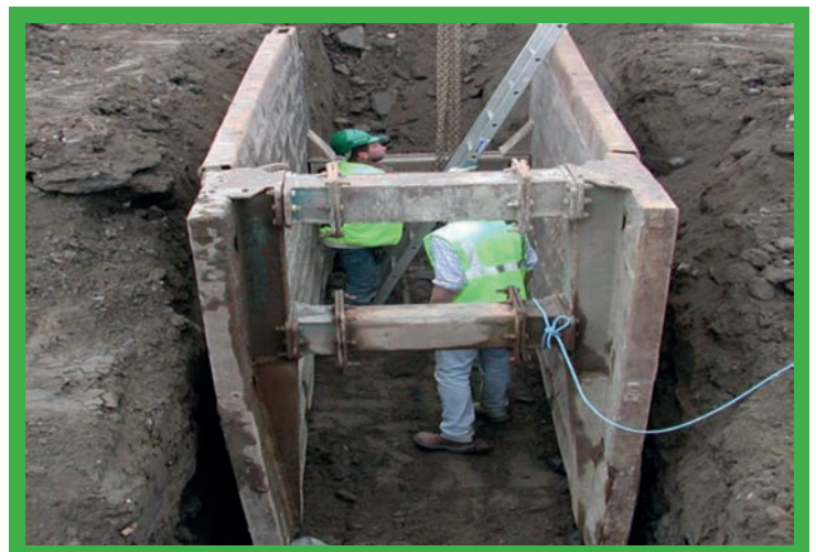
Trench Boxes in use.
