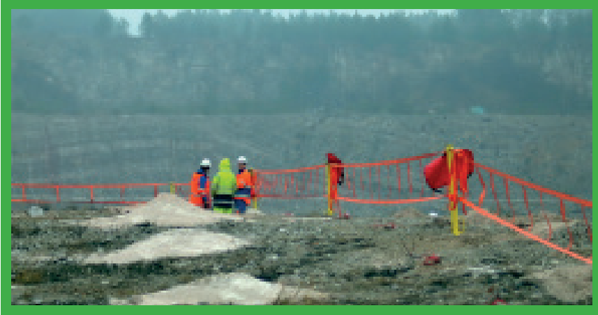
Barrier system at quarry face.
