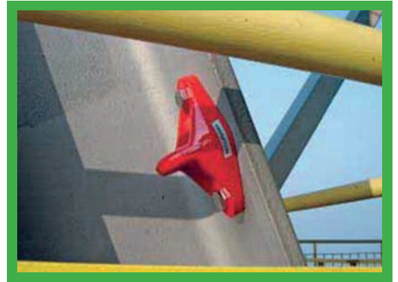
Additional securing hooks for harness use - installed where required.
